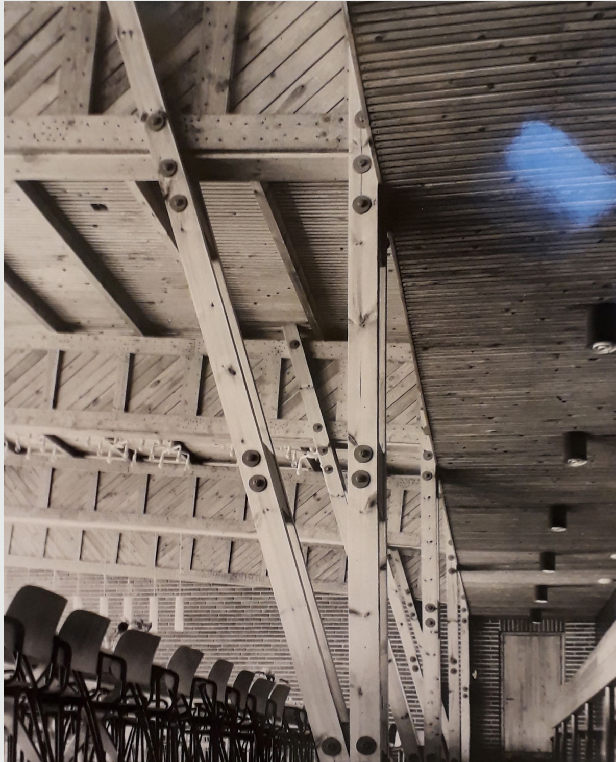
Servin mökin nailed truss from timber pieces
