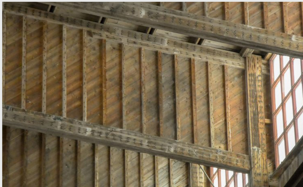
apx. 35m span nailed truss from reclaimed timber pieces
