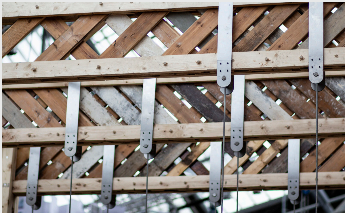
Structurally optimized beam system from reclaimed timber pieces
